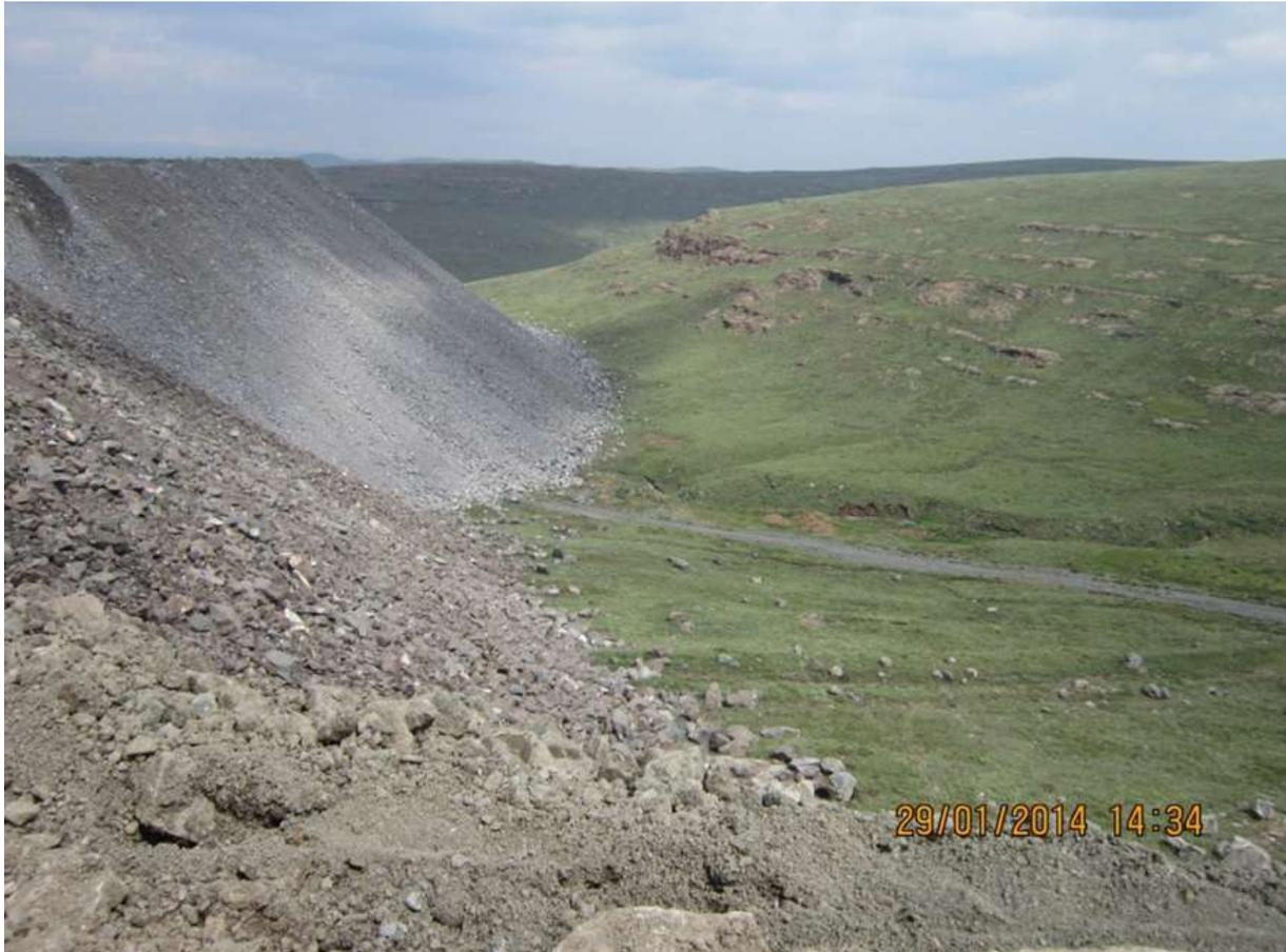
*Figure 10. Oversize material segregates down to the toe of the waste rock dump.*
